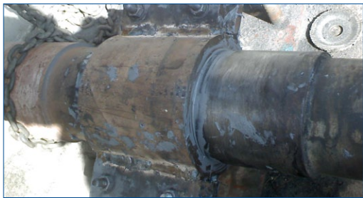
Belzona applied, former in place
