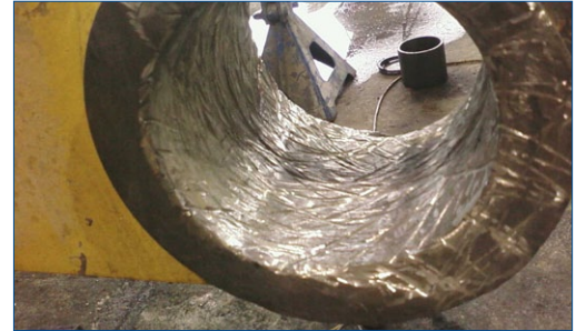
Surface preparation completed
